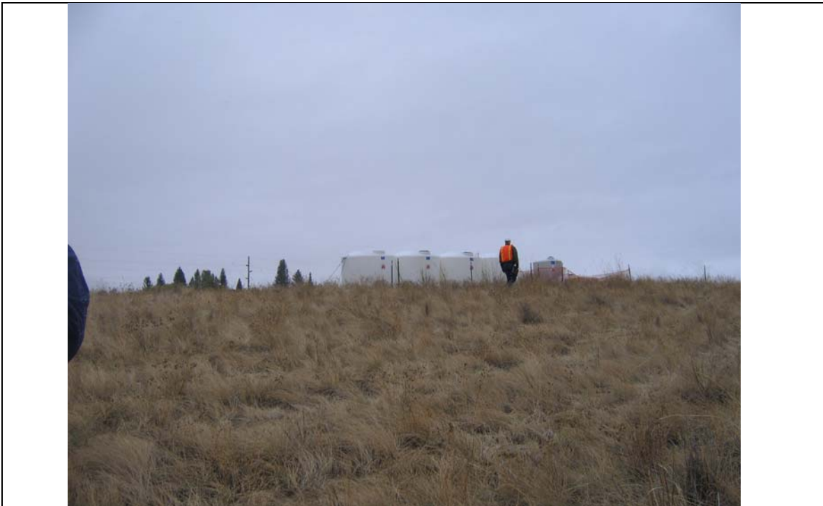
Photo 7. Empty tanks (used for previous groundwater dosing)
