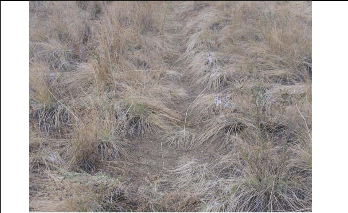
Photo 9. Tire ruts from repeated driving on repository cap.
