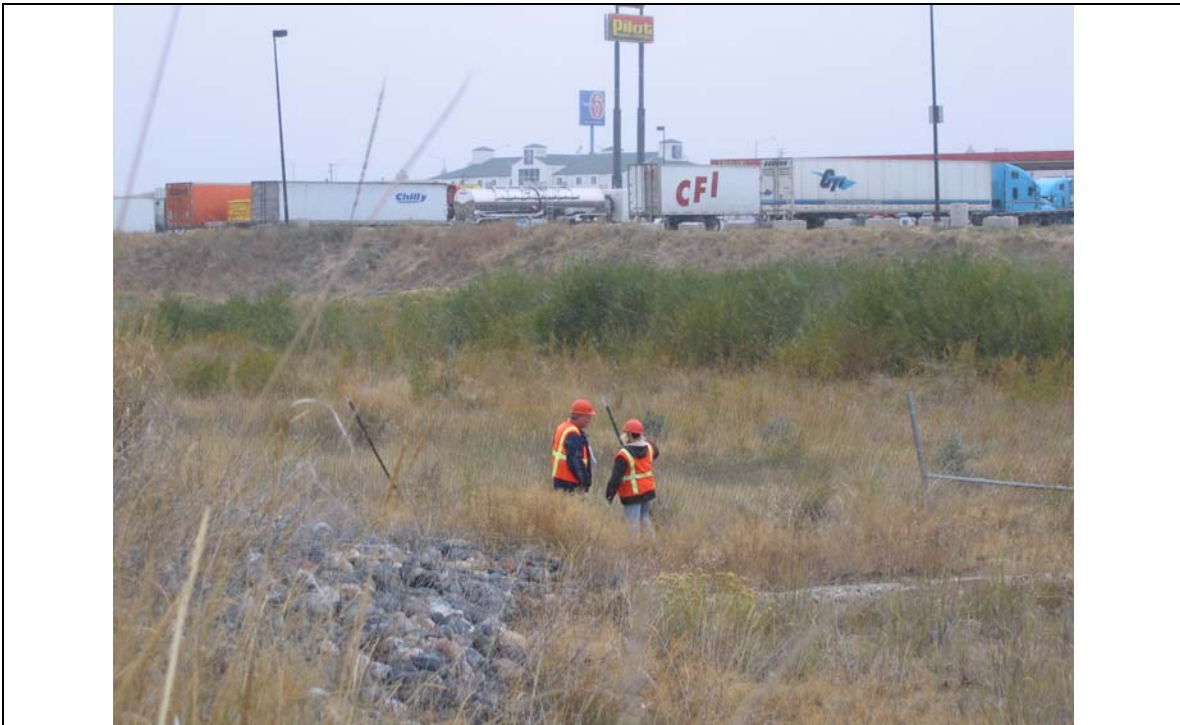
Photo 5. Damaged fencing along edge of repository. Rip rap visible in foreground.
