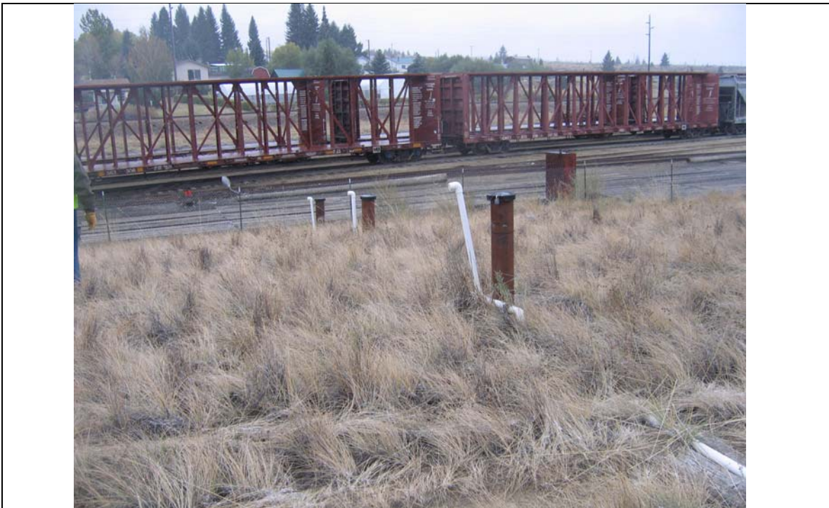
Photo 8. Array of injection wells remaining from groundwater dosing.
