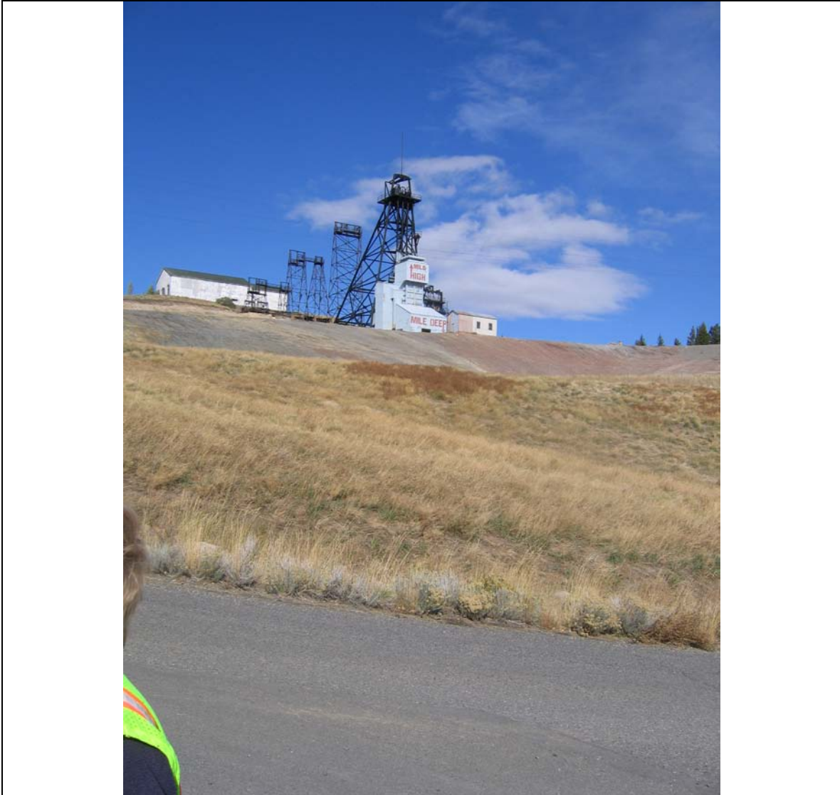
Photo 7. Mountain Con headframe and recontoured waste dump with Little Minah dump reclamation in the foreground.
