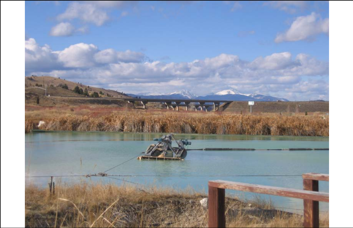
Photo 3. Lower Area One B1 Cell Sludge Dredging Barge
