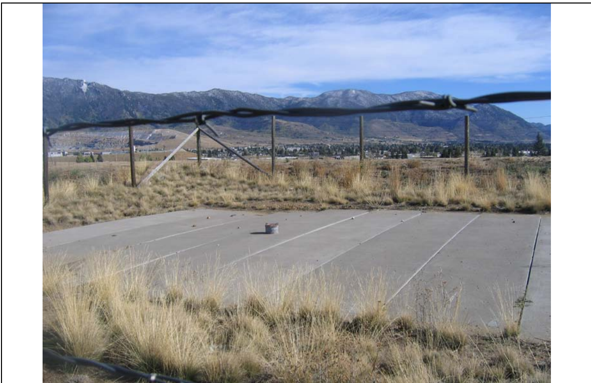
Photo 9. Concrete Cover over the Otisco Shaft
