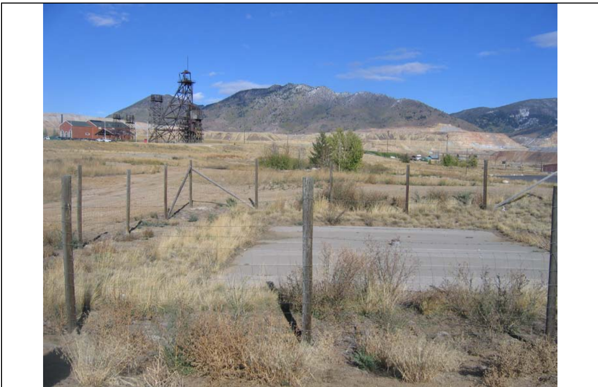
Photo 11. Looking Northeast over the Otisco shaft cover.
