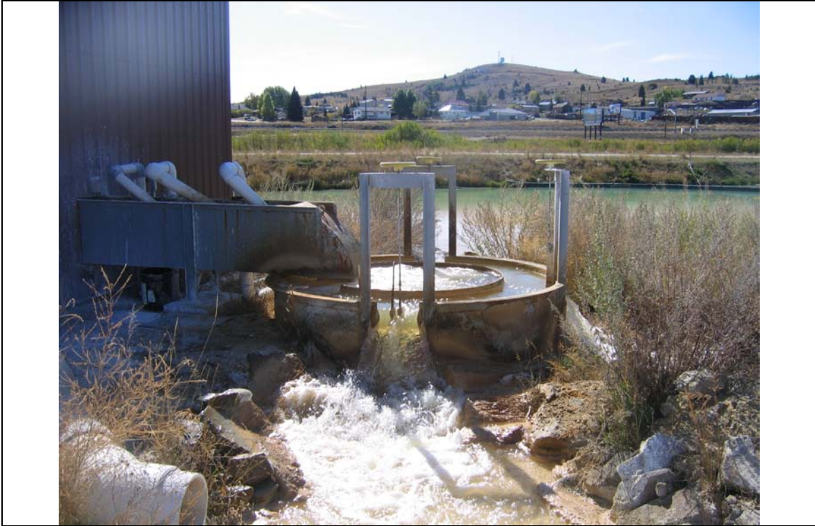
Photo 1. Lower Area One Flow Distributor
