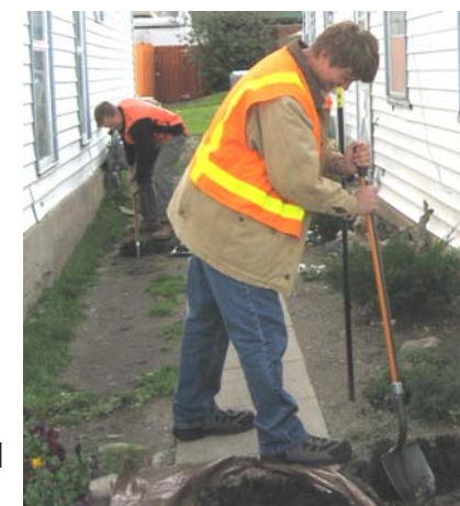
2007 subsurface yard sampling
