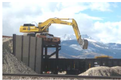
Excavator unloading rail cars
