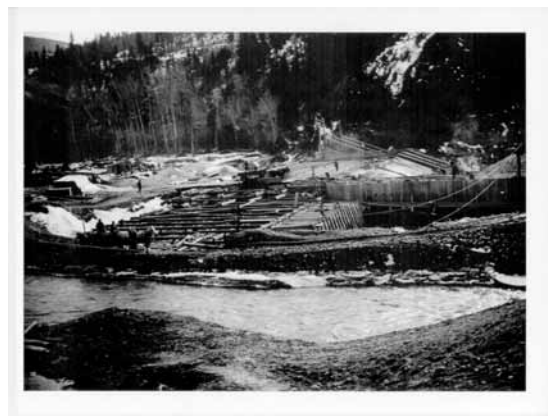
Milltown Dam Construction, 1906
