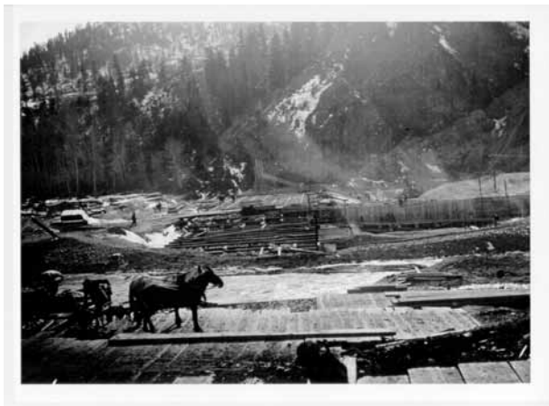
Milltown Dam Construction, 1906
