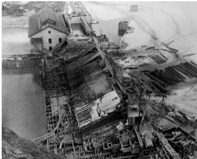
Reconstruction of Milltown Dam following 1908 flood
