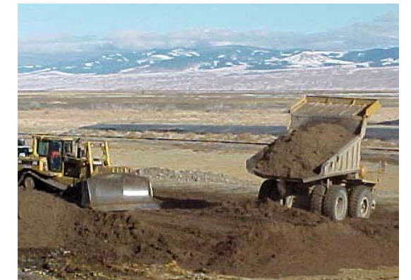
Placing Cover Soil
