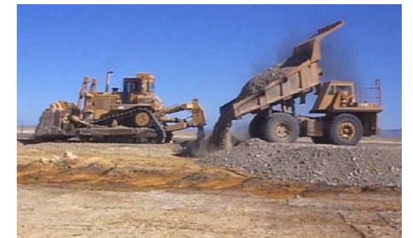
Building haul roads and spreading cover
