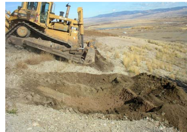
Constructing dozer basins
