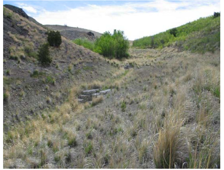
Photograph 5722. Some open ground but good overall perennial vegetation cover in Nazer Gulch. Gabion rock dropped structures are intact and functional. Work conducted under RDU 3 – Anaconda Ponds WMA.
