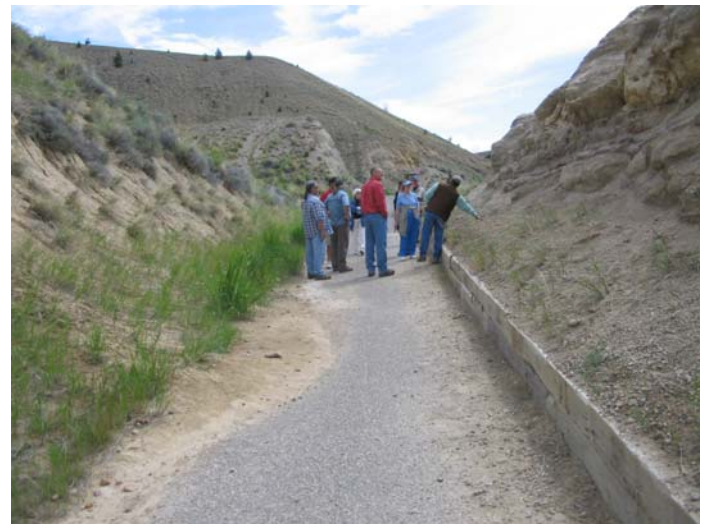
Photograph 5834. Sediment discharging onto the historic trail.
