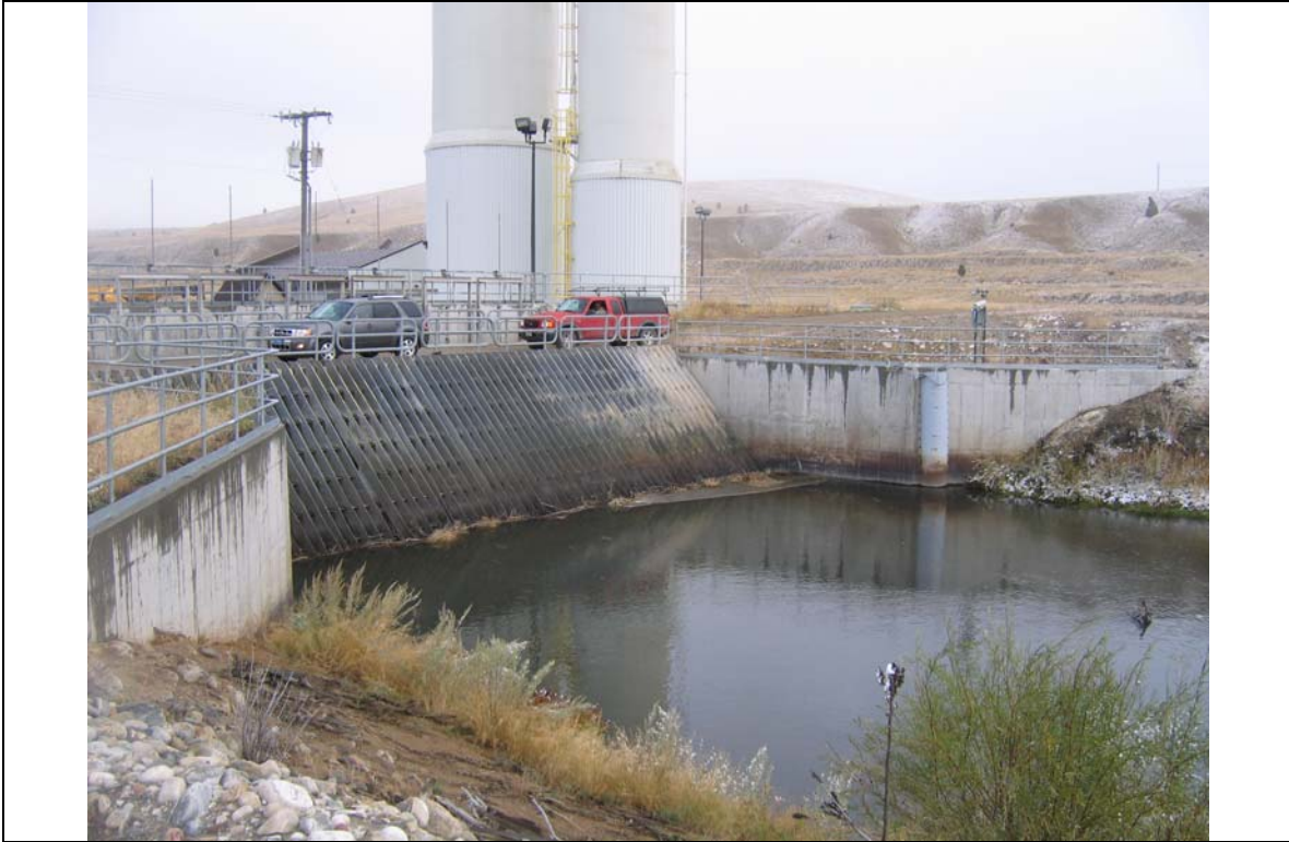
Photo 1. Silver Bow Creek entering the WSP hydraulic control structure and trash racks. Lime silos in background center.
