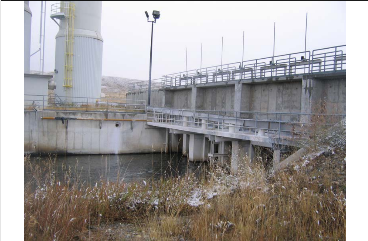
Photo 2. Downstream side of the WSP hydraulic control structure with lime silo towers in background left.
